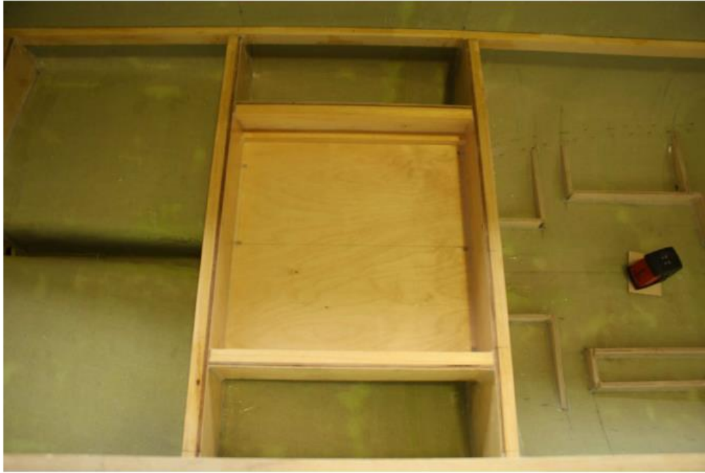
Figure 11: Void 8; engine & electric workshop etc. (#39 to #60)
