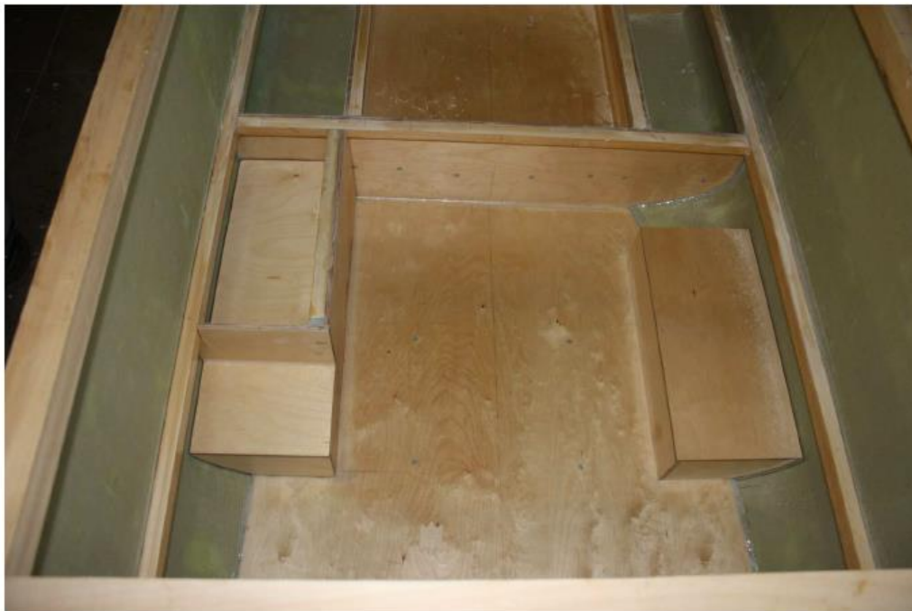
Figure 15: Engine room; void 7; purifier plant 2
