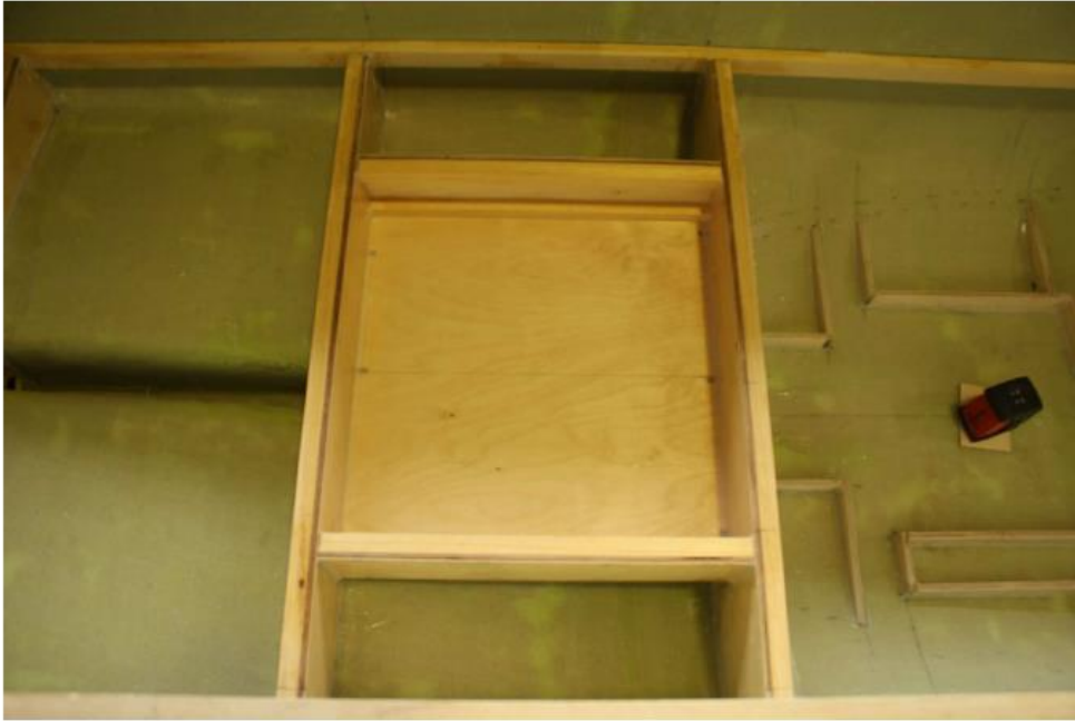
Figure 11: Void 8; engine & electric workshop etc. (#39 to #60)
