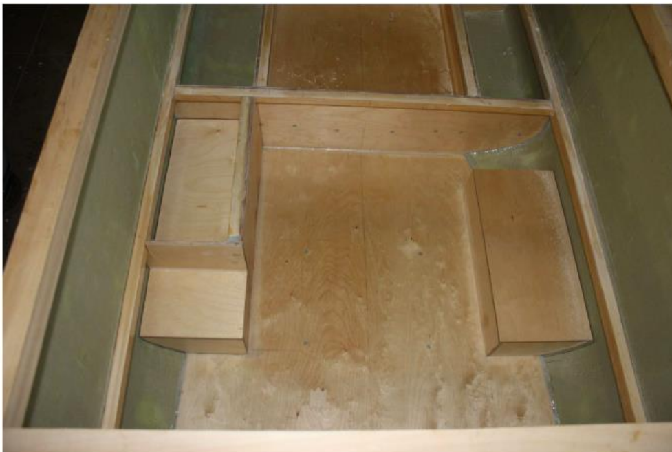
Figure 15: Engine room; void 7; purifier plant 2
