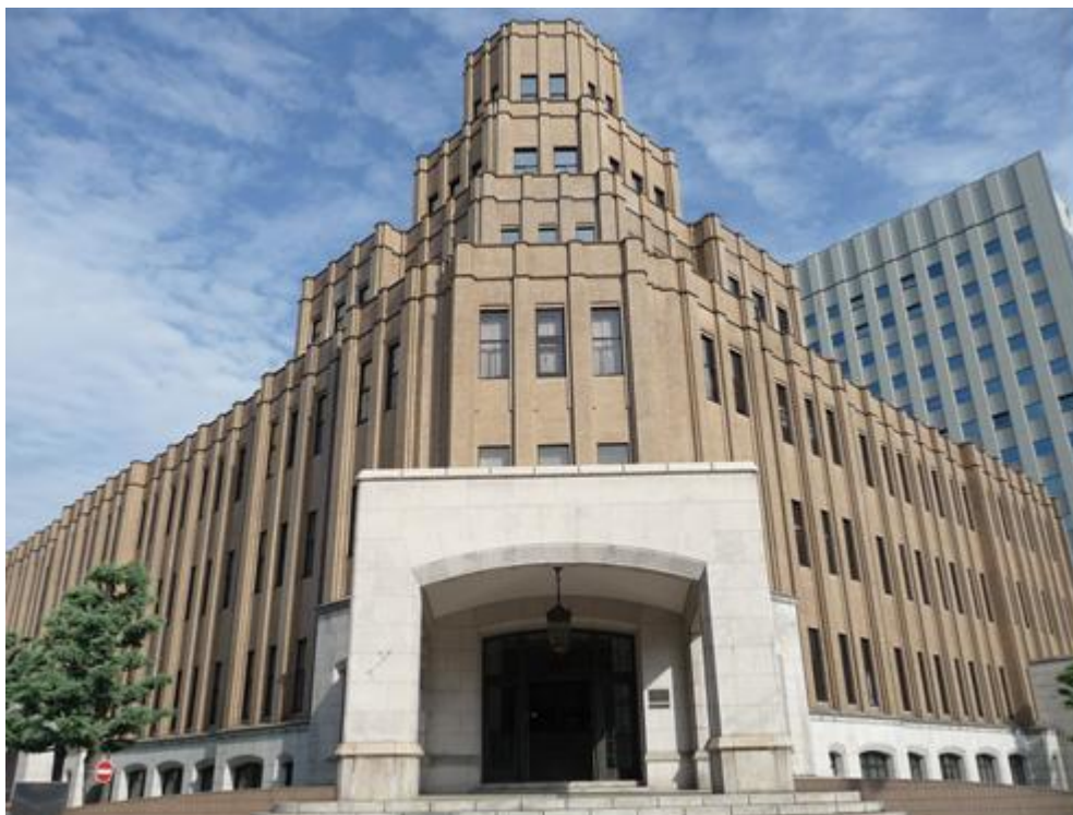
The Courthouse of Fukui District Court
